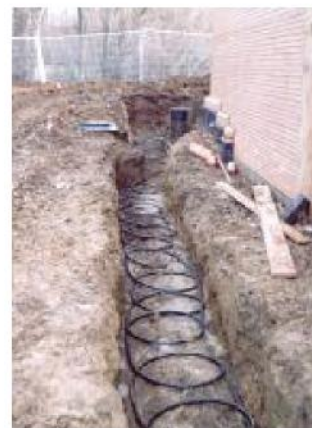
The 'slinky' ground loop being installed in a trench at the National Energy Foundation
