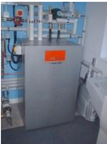
The Heat Pump in the new offices at The National Energy Foundation
